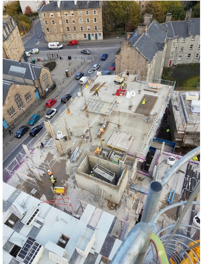
View from Tower crane to Bernard Terrace
